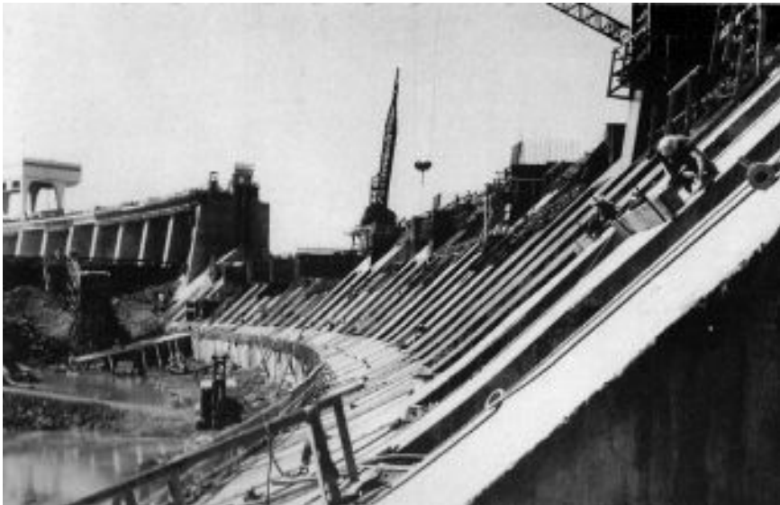
THIS IS THE LONG SAULT RAPIDS AREA AFTER IT WAS DRIED UP. NOTE THE TOWER IN BACKGROUND THIS WAS PART OF THE COPPER DAM USED TO DRY UP THE WATER.
